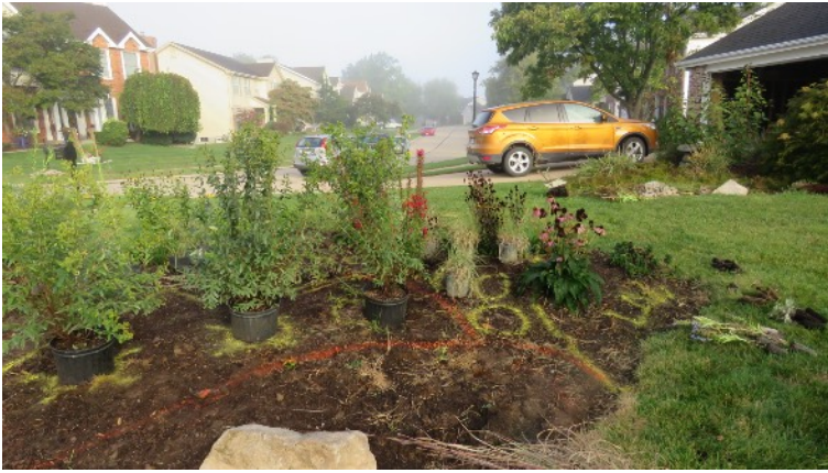
Designated areas were outlined for the places where the new plantings will go.
